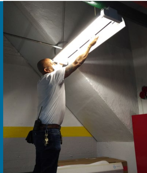
The Fireman at The Christa McAuliffe School in Brooklyn installs a lighting upgrade.
