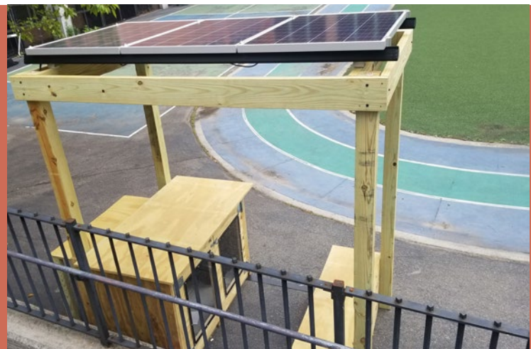
A Demonstration Solar Installation (Trellis Design) at Central Park East, Manhattan.
