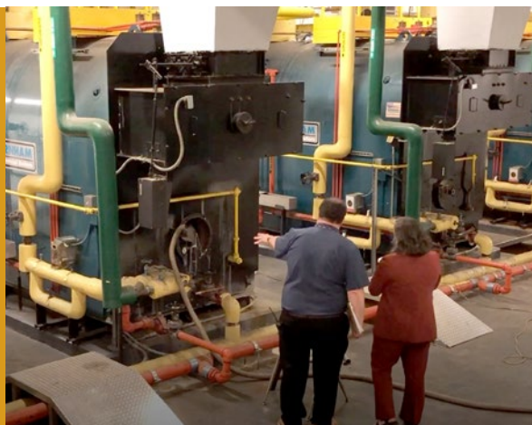
Custodian Engineer Anthony Delrosso gives a tour of the boiler room at Boys & Girls High School, Brooklyn.
