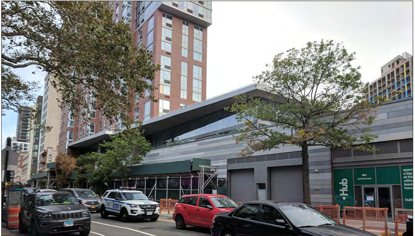
The one- to three-story base of 333 Schermerhorn Street. View from Schermerhorn Street west of 3rd Avenue facing northwest. 15
