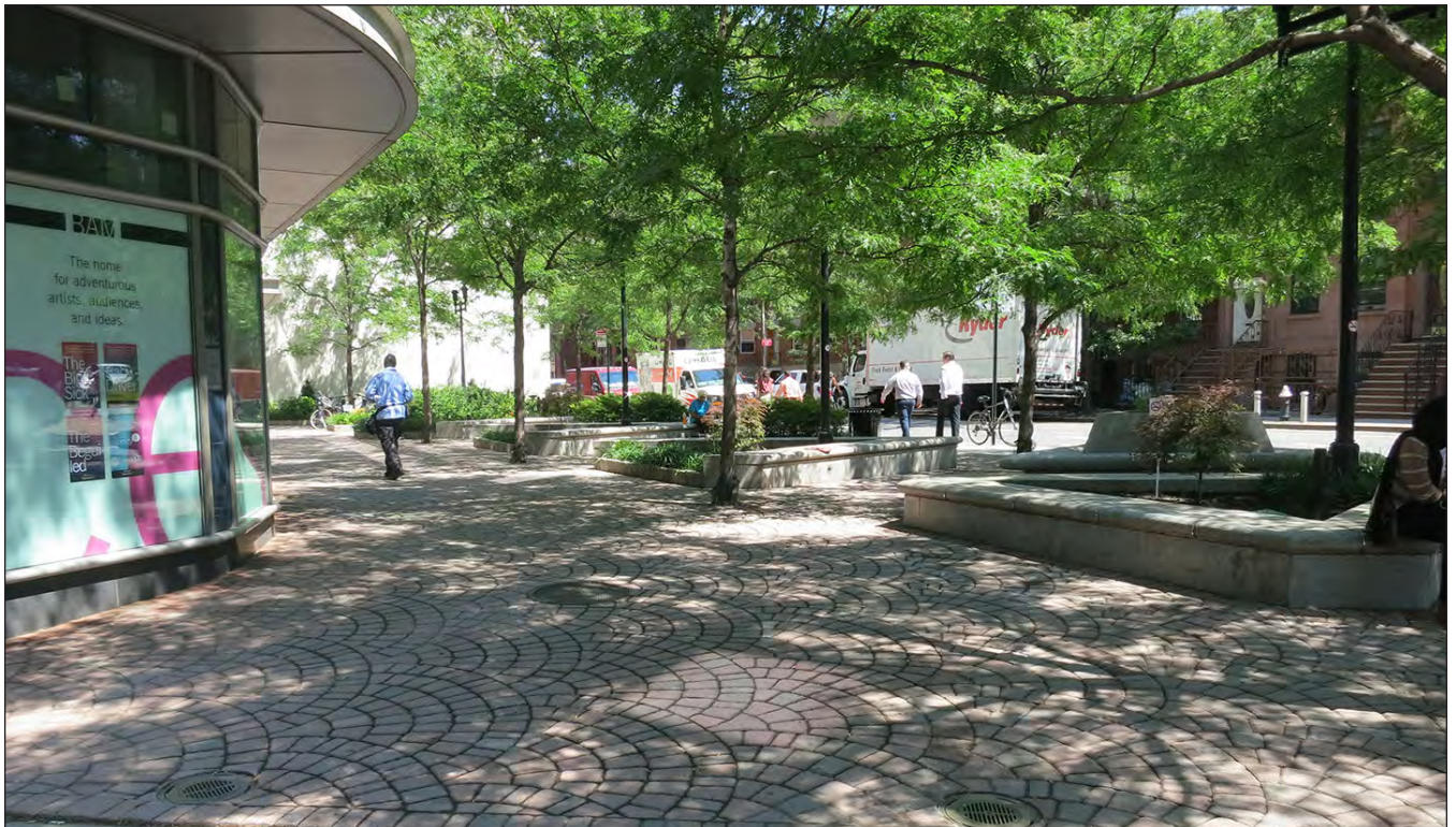
The plaza at Ashland Place and Fulton Street contains planting beds, benches, trees, lighting, and decorative pavers. View from Fulton Street facing northeast. 30
